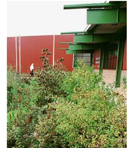
Runoff conveyed into planter
