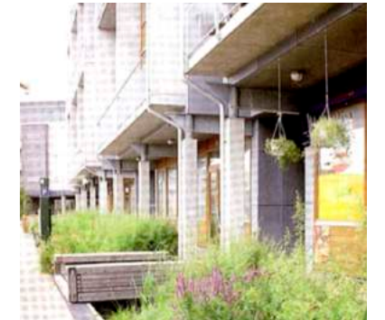
Roof water conveyance
