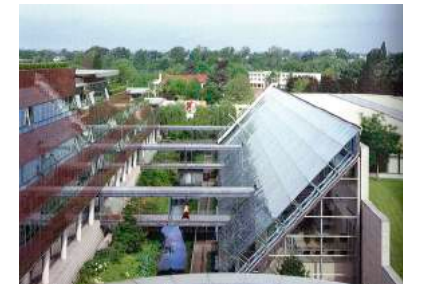
Architectural connections between old and new buildings
