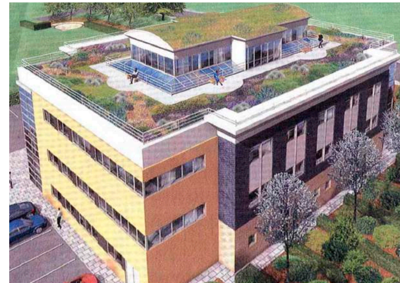
Green roof with usable pathways and seating
