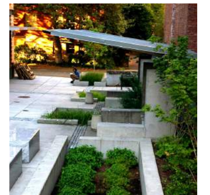
Water collected from canopy is conveyed into planter
