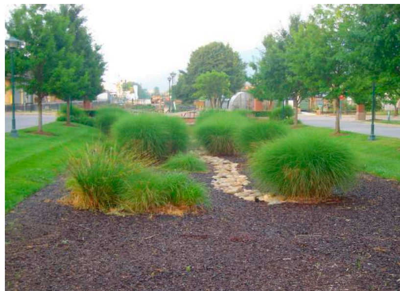
GREEN STREETS Less developed streets, shown here with a bio-swale
