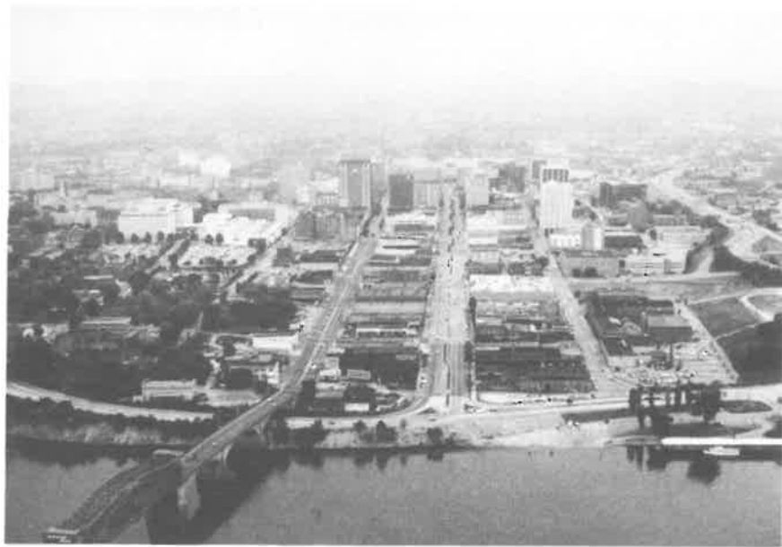
Existing Conditions at River's Bend
