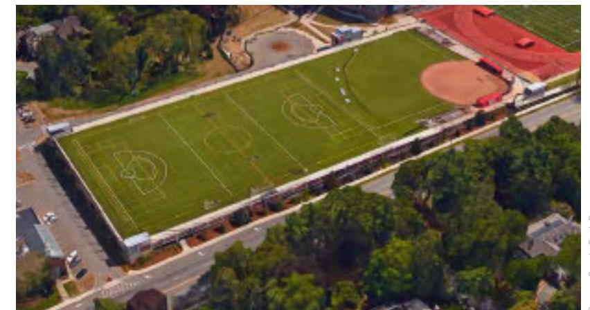
Precedent at Worcester Polytechnic Institute in Worcester, Massachusetts
