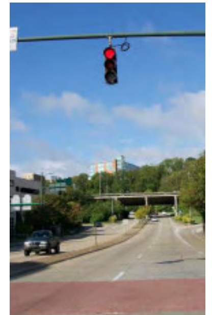
4th Street at the highway 27 interchange
